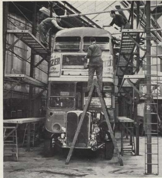
Fig. 3 Special gantries in the paint preparation shop
